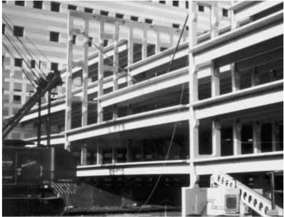
Figure 7-3 Braced "lite walls" during erection.
