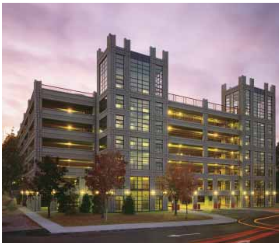
Boston College Parking Structure, Chestnut Hill, MA
