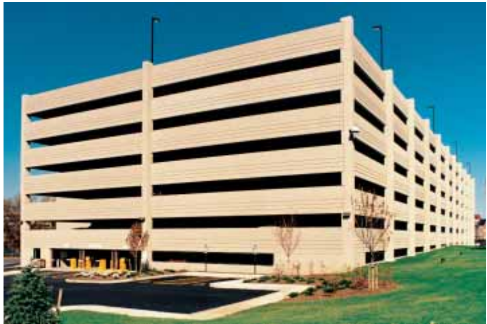
Station Plaza Parking Garage, Trenton, NJ
