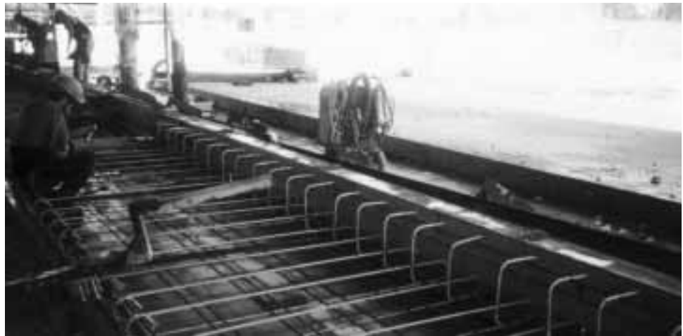
Figure 6-1 Ledged spandrel in form.
