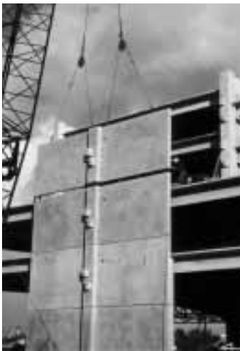
Figure 7-4 Story height wall panels "Stacked."
