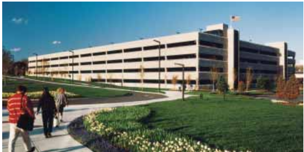
Pfizer Inc. Parking Structure (Building 290), Groton, CT
