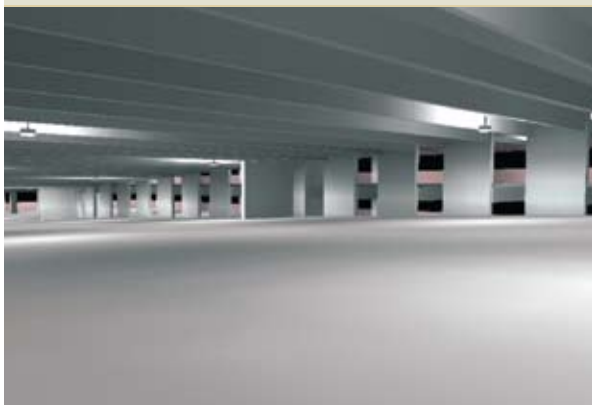
Figure 3. The interior of a precast concrete parking structure is used for illuminance comparison.
