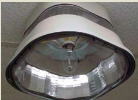
Figure 7. A Gardco GP1 luminaire can be used for lighting in precast and post-tensioned concrete parking structures.
