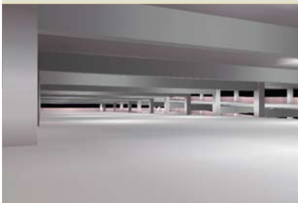
Figure 4. The interior of a post-tensioned parking structure is used for illuminance comparison.
