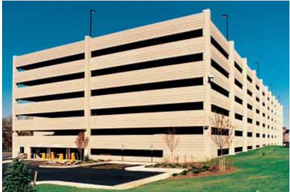
Station Plaza Parking Garage, Trenton, NJ
