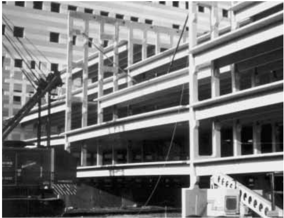
Figure 7-3 Braced "lite walls" during erection.
