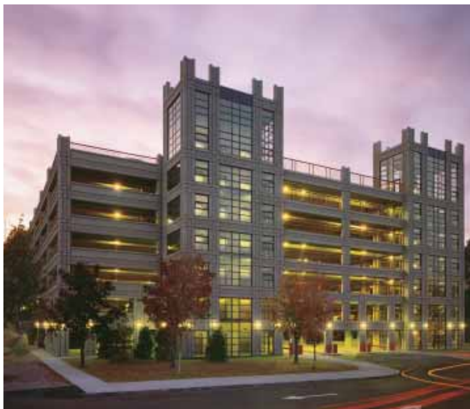
Boston College Parking Structure, Chestnut Hill, MA
