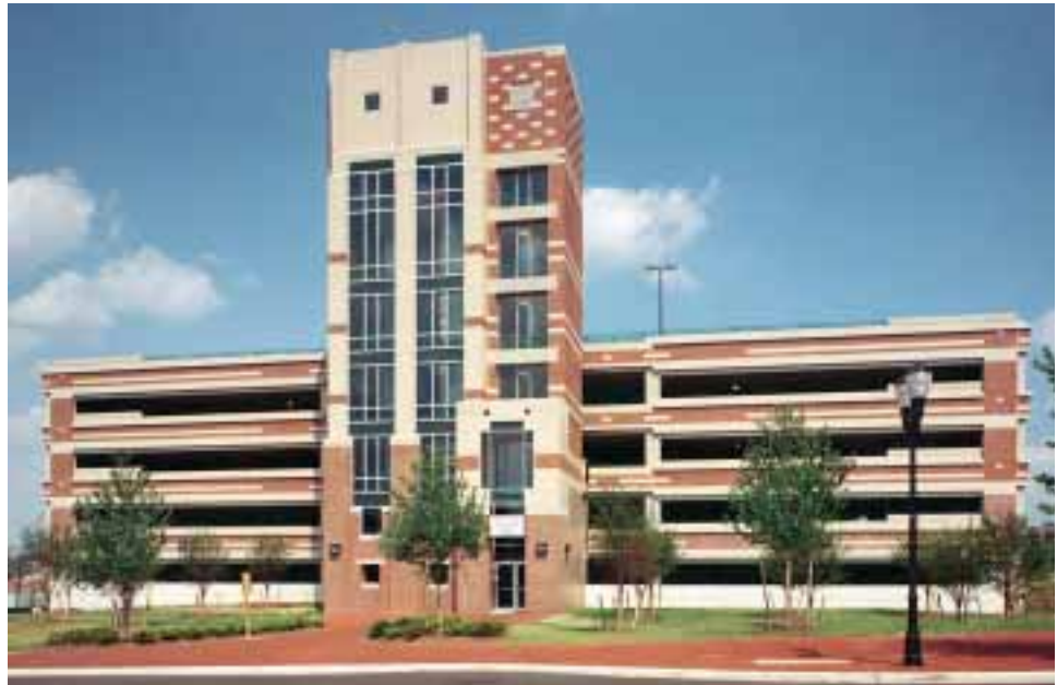
Camden Waterfront Parking Garage, Camden, NJ
