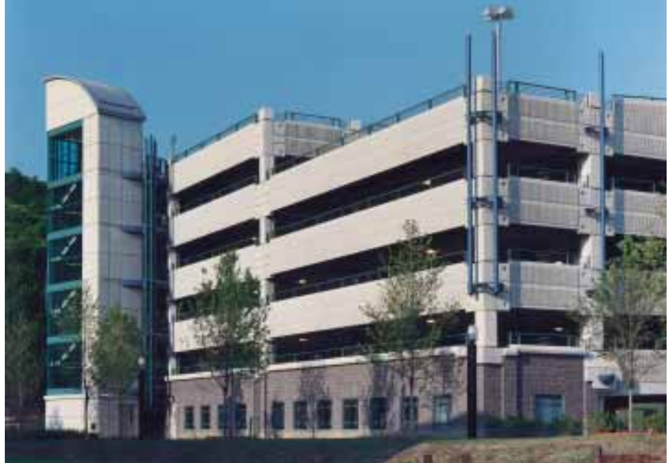
Pittsburg Technology Center Garage, Pittsburg, PA
