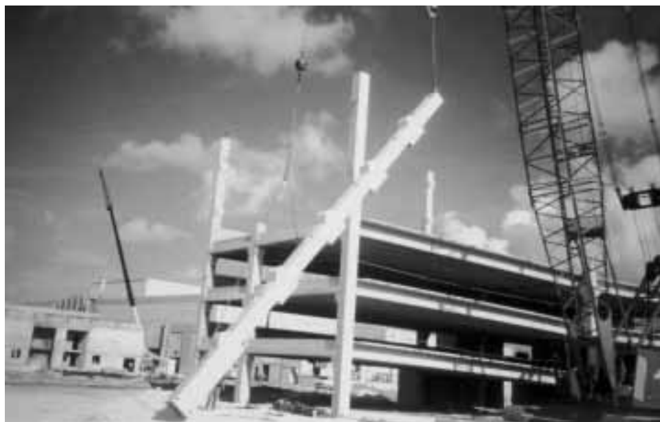
Figure 7-2 Rotating a column into position.
