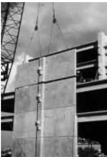
Figure 7-4 Story height wall panels "Stacked."
