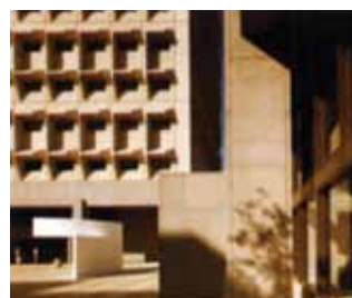
Figure 11 Deep recessed windows and overhang (eggcrate device). (Courtesy © MBA)
