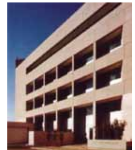
Figure 10 Deep recessed windows. (Courtesy © Glen Allison)
