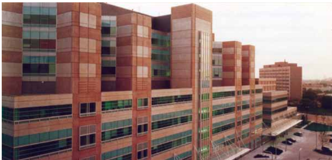
Figure 36 Insulated sandwich wall panels. John H. Stroger, Jr. Hospital of Cook County, Chicago, Ill. CCH Design Group headed by Loeb Schlossman & Hackl. (Courtesy ©Hedrick Blessing)
