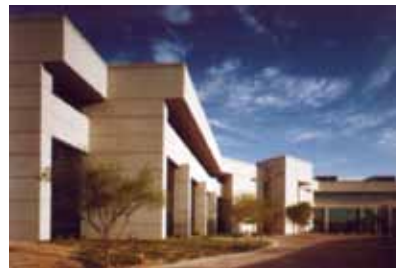
Figure 9 Cantilevered floor used to shade windows.
